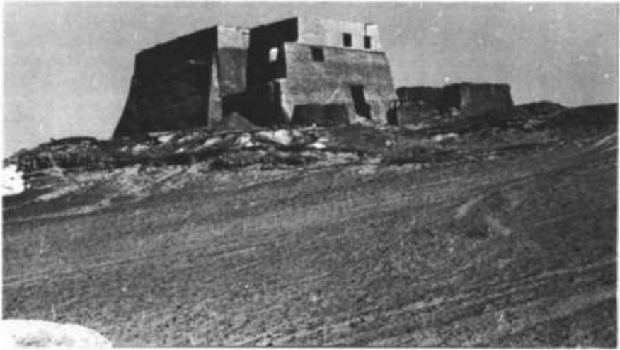
PLATE 8.1 The royal building in Old Dongola, converted to a mosque in 1317
