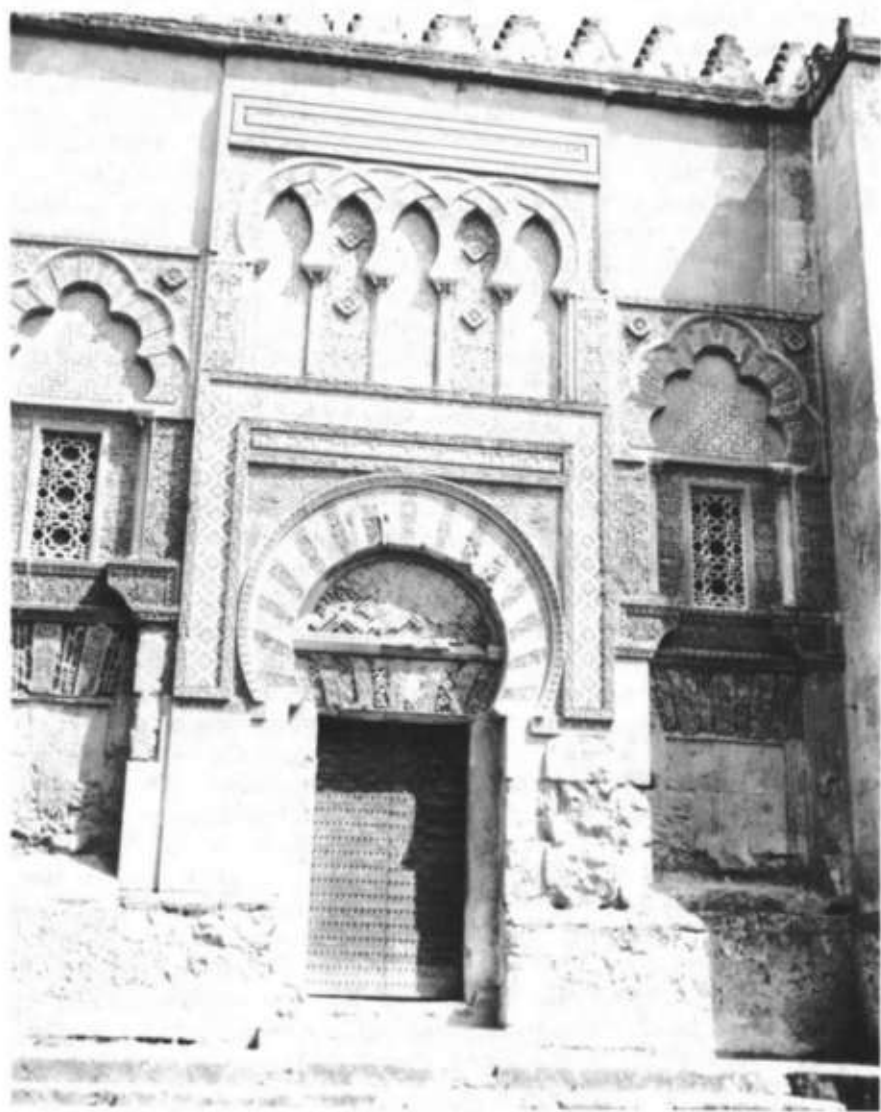
PLATE 10.6 Door and blind arches of the west façade of the mosque at Cordoba
