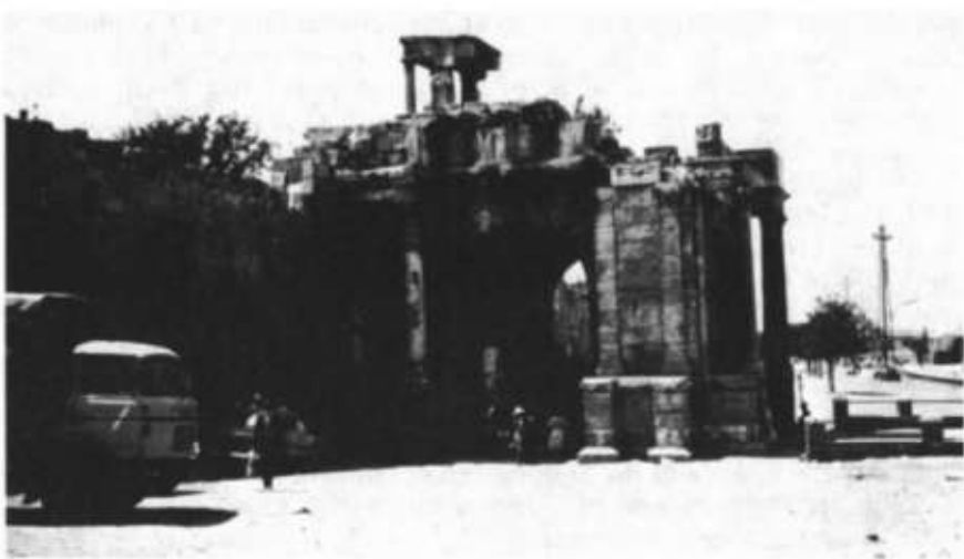
PLATE 9.1 Part of the Byzantine fortifications of the city of Tebessa: Arch of Caracalla, originally in the centre of the Roman city, converted by the Byzantines into the north gate of a much smaller, walled town eventually conquered by the Arabs.
