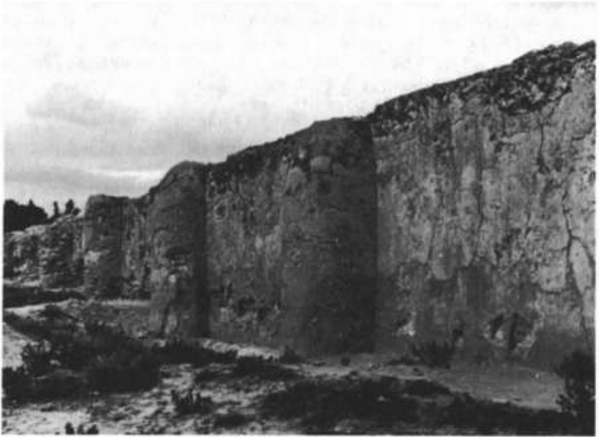
PLATE 10.5 The great lake of Raḳḳāda, near Ḳayrawān. Massive embankments served as a breakwater against waves whipped up by the wind
